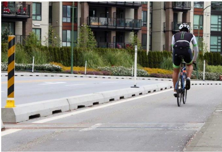
Pre-cast curb-height concrete barrier
