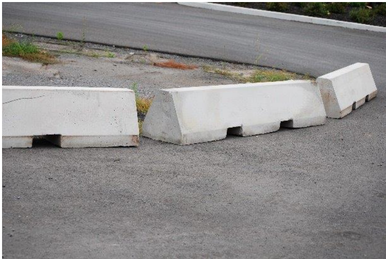
Mid-height concrete barrier
