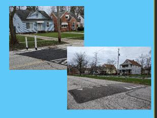
Formed asphalt speed tables with associated signage, curbside delineators, and roadway striping
