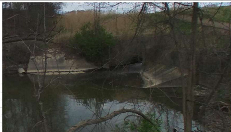
Dam Primary Outlet Plunge Pool Rock Lining
