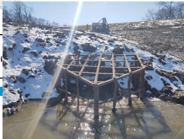
Dam High & Low-Level Trash Rack Modifications
