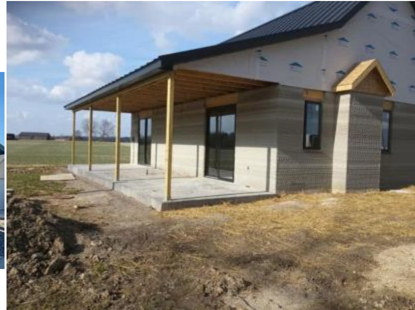
Sustainable Concrete Solutions
