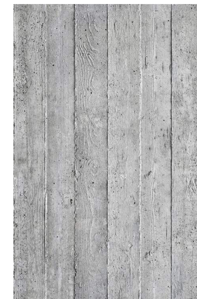
BOARD FORMED CONCRETE CONC-1
