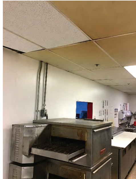
A12 - Finish ceiling in kitchen area
