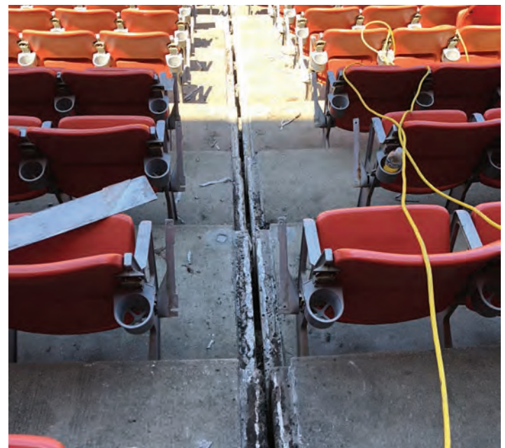
S7 - Typical Precast Joint
