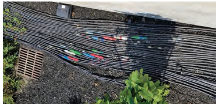
E15 - Temporary power cables laid on ground - north side
