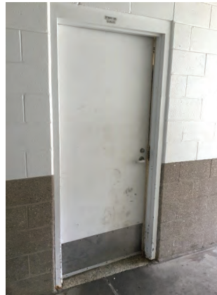
A3 - Typical hollow metal door assembly
