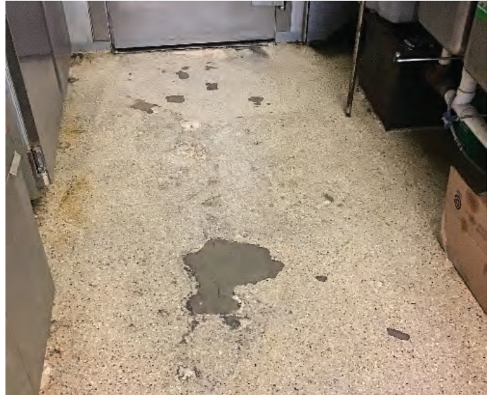
A11 - Epoxy floor in kitchen area
