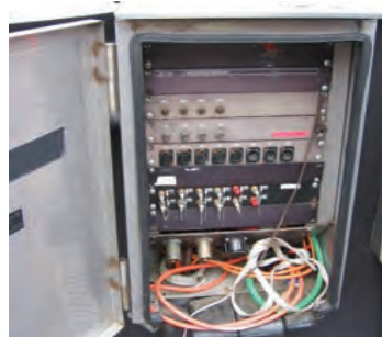
T1B - Internal View
