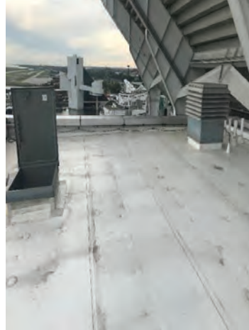
A1 - Typical single-ply membrane roof
