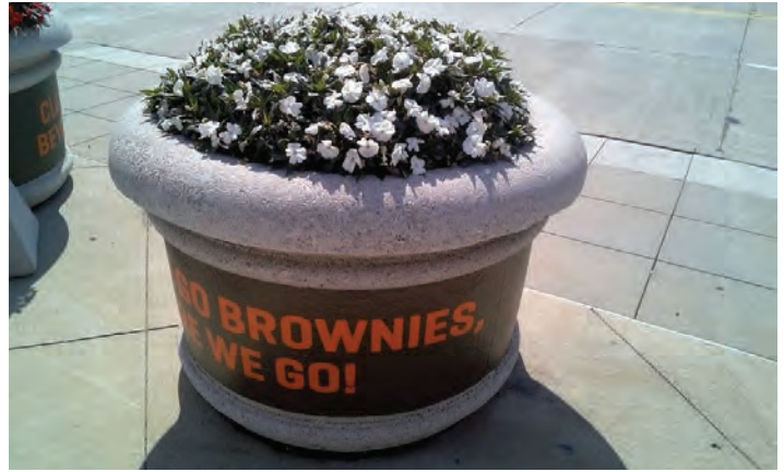
L5 - Precast concrete planter bed
