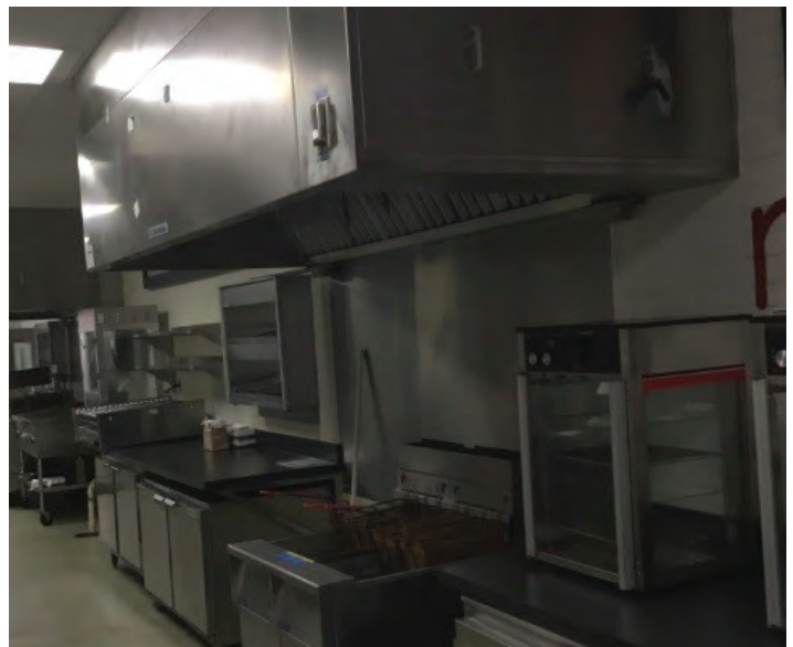
M5 - Typical Concession Exhaust Hood
