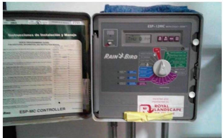
L7 - Existing irrigation controller
