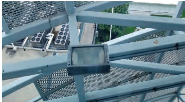
E10 - HID fixture mounted behind windscreen
