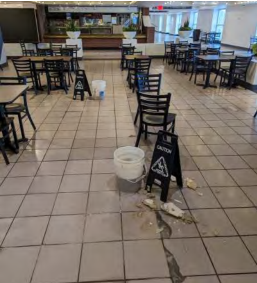
Deteriorating floors, walls, and stairwell in the Tower City building associated with Raisin Industry Parcels
