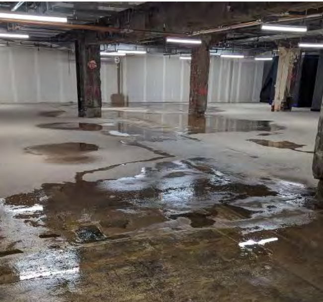
Poor ventilation highlighted by damp conditions and standing water causes paint to peel and fosters the growth of mold and mildew associated with Raisin Industry Parcels.
