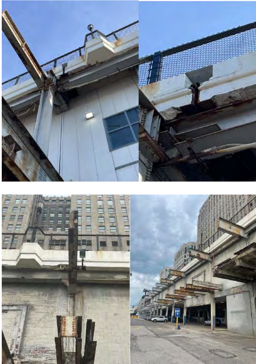
Deteriorating beams, parapet, and crumbling concrete on the exterior of Raisin Industries parcels.
