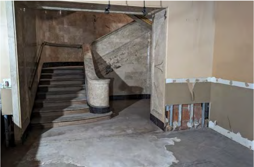
Deteriorating floors, walls, and stairwell in the Tower City building associated with Raisin Industry Parcels
