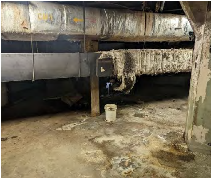
Poor ventilation highlighted by damp conditions and standing water causes paint to peel and fosters the growth of mold and mildew associated with Raisin Industry Parcels.
