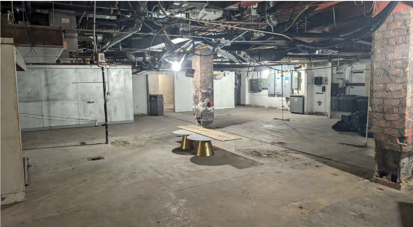
Exposed overhead wires, dilapidated flooring, and crumbling brick associated with Raisin Industry Parcels.
