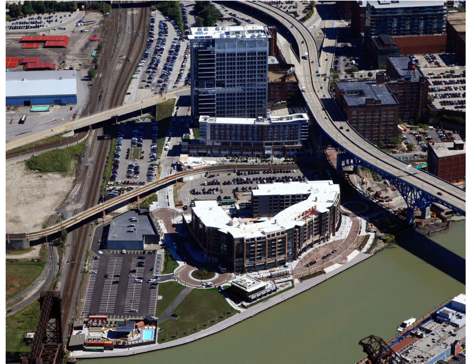
COMPLETED PHASE I AND 2
