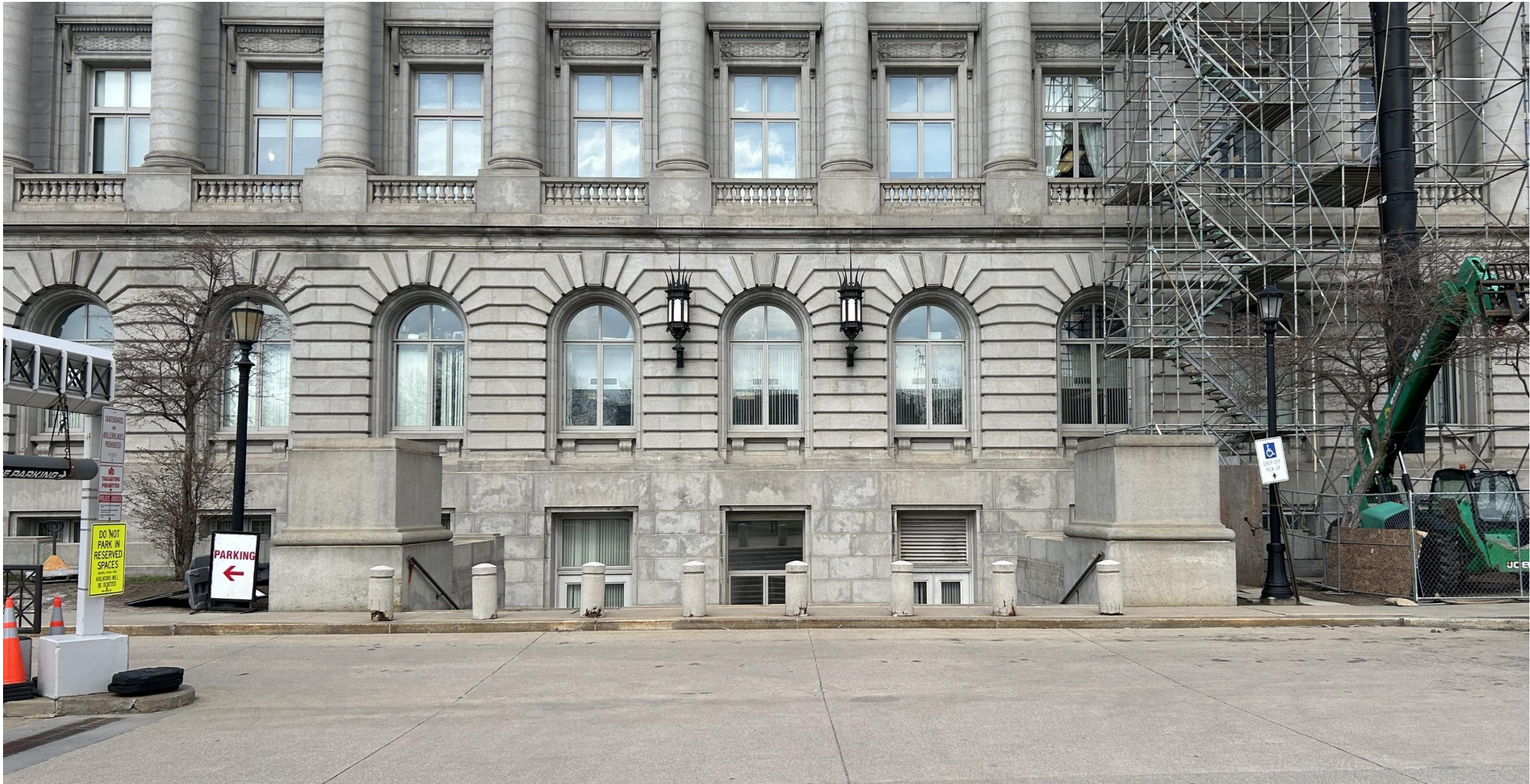
WEST DOORS (FORMER ENTRANCE) EXISTING CONDITIONS
