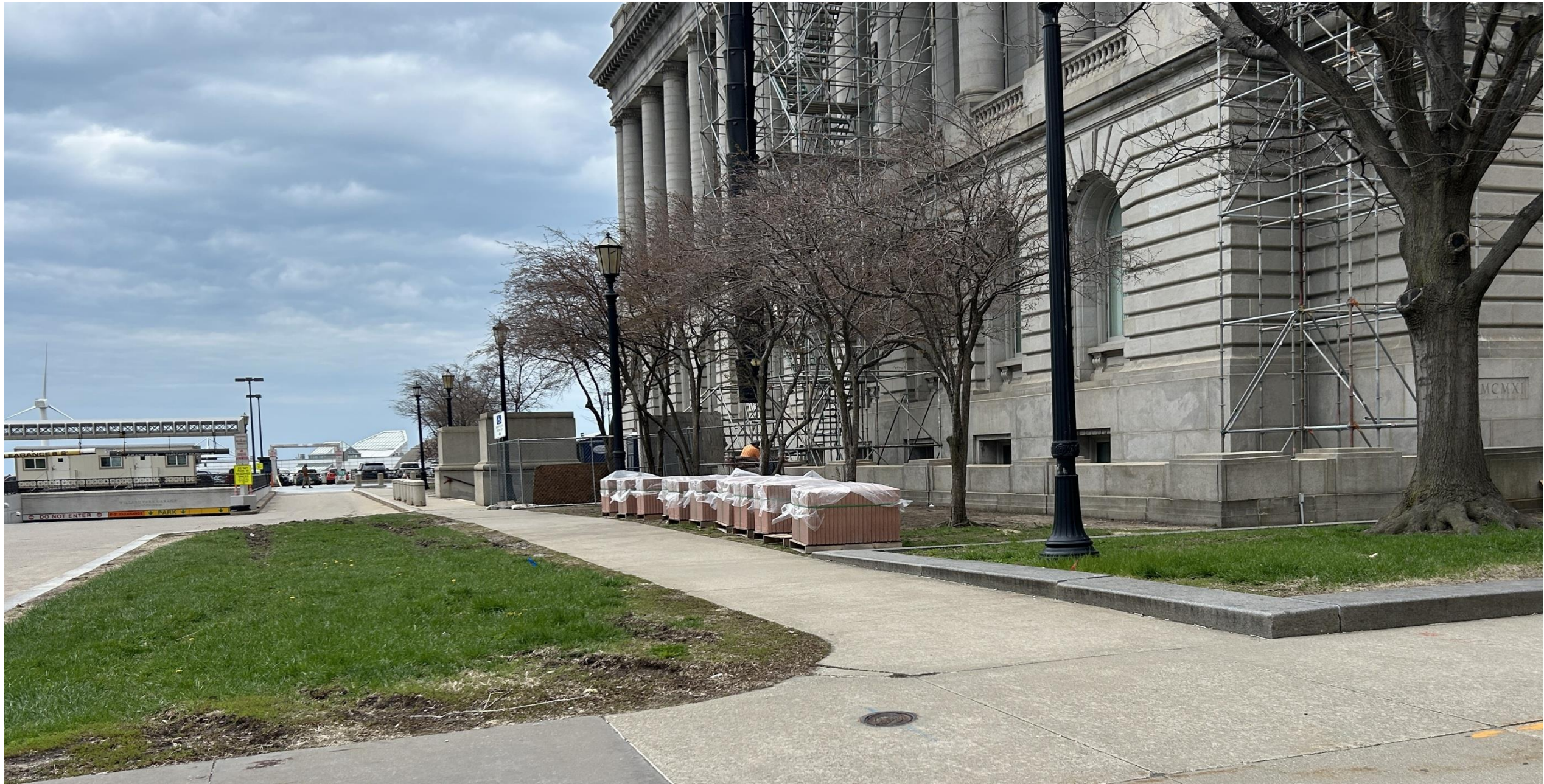
WEST ENTRANCE RAMP EXISTING CONDITIONS
