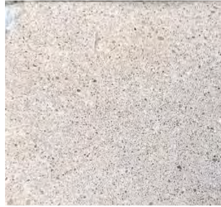
Sculpture Base Cast in Place Concrete (Sandstone Color)
