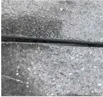
Donor Wall Polished Cast in Place Concrete (Medium Gray Color)
