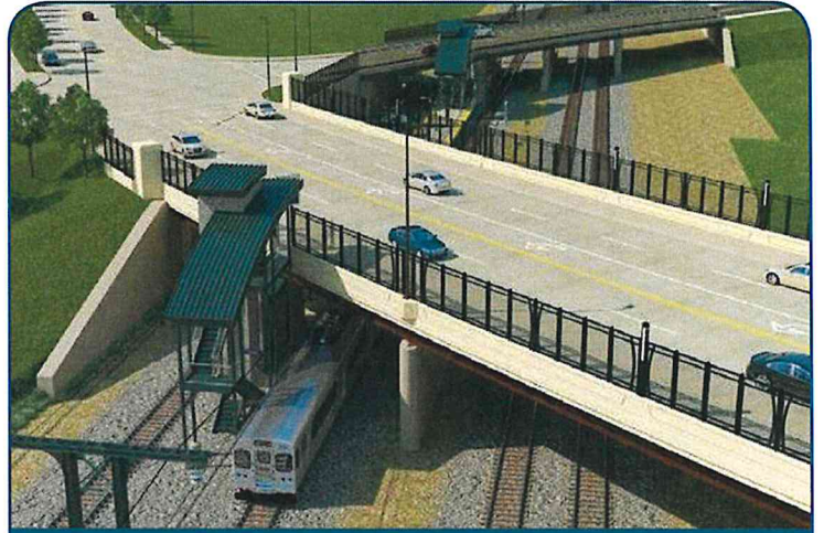
The Greater Cleveland Regional Authority's investment in the Quincy - E 105th St Station demonstrates a commitment to retaining and enhancing increased transit access to the Innovation Square neighborhood. Image courtesy of GCRTA.
