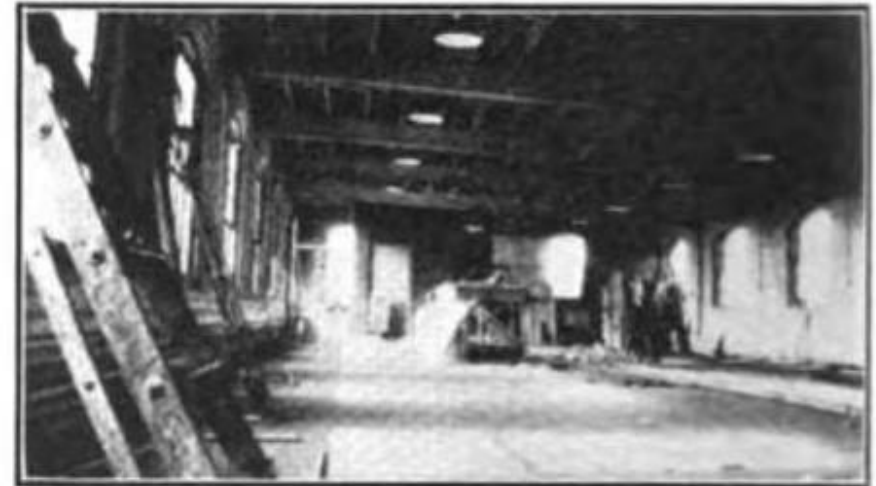
Inside of Laboratory from North End Showing Supervisor's Office.
