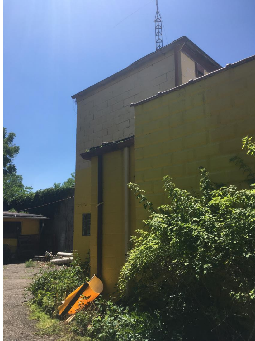
Rear part of studio, east side
