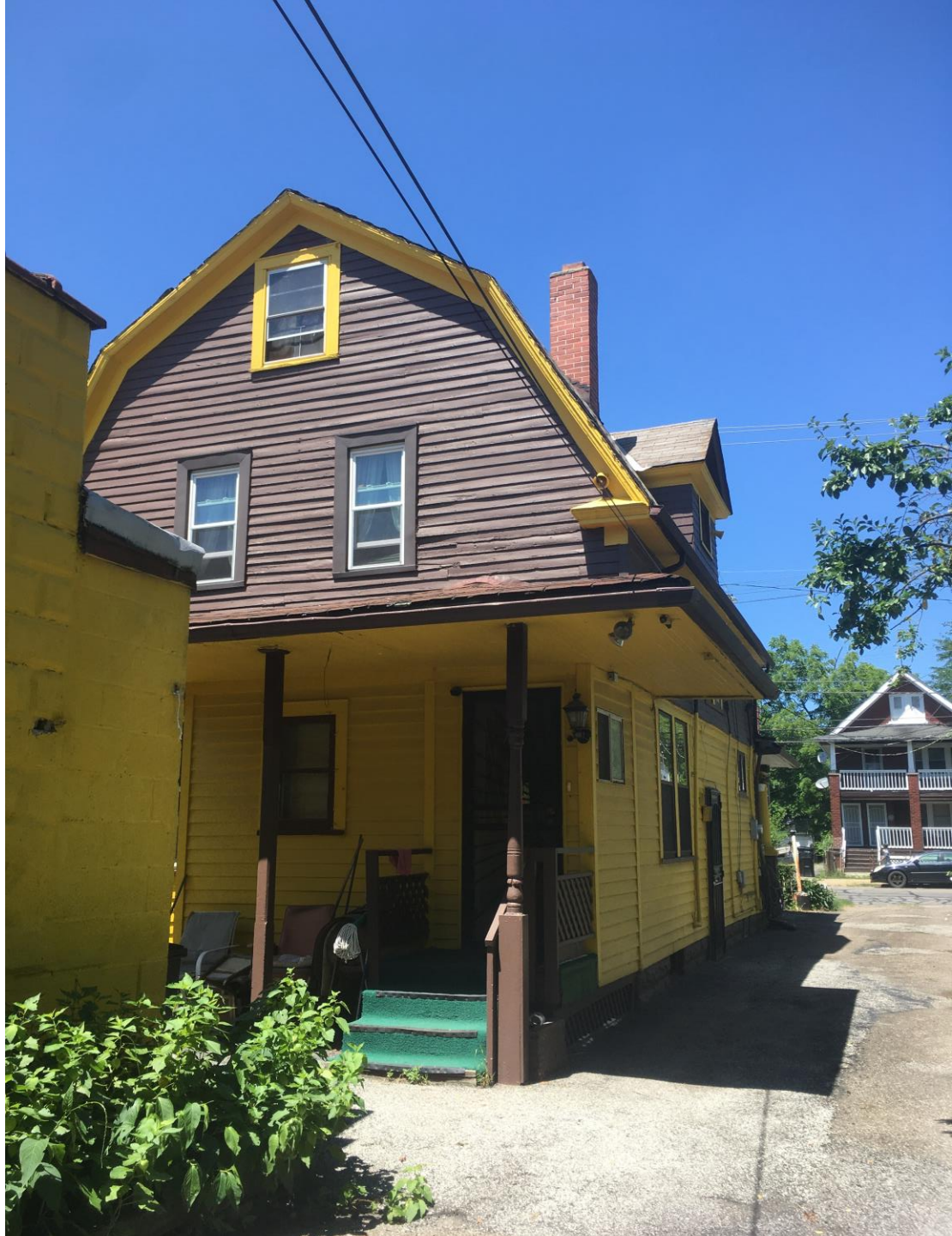
Back of the house, east façade, corner of studio, view down the driveway (PC: Julia LaPlaca, July 2020)
