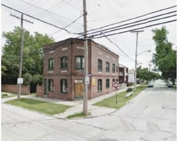
Intersection of West 58th and Herman Avenue
